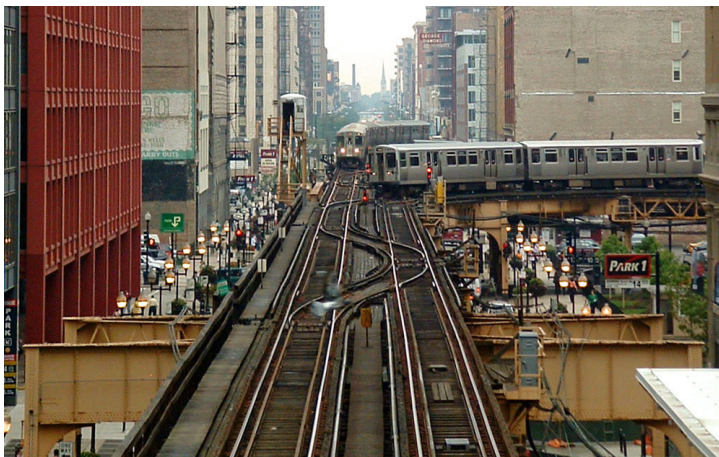
Figure 6.13. Chicago 'L' light rail
