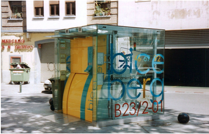
Figure 6.17. Biceberg is an automated underground bicycle parking system in Zaragoza, storage for 46 bicycles
